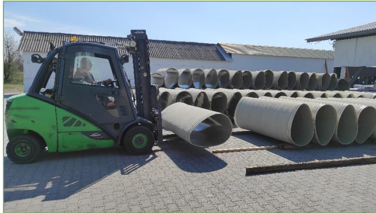
Figure 6: Moving with forklift
