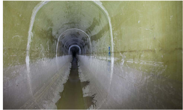
Sewer lining by oval GRP pipes
