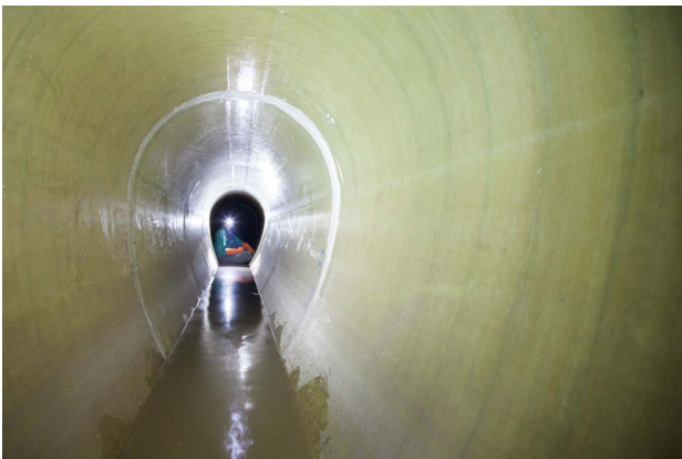
Pipelining by GRP pipes of egg-shape
