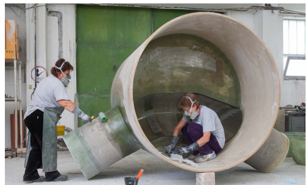
Manufacturing of a cleaning shaft for waste water
