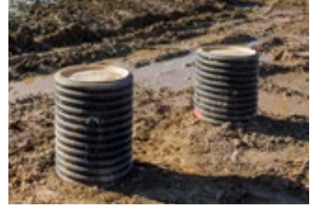
Temporary construction site cover for extension pipes
