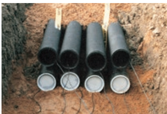
Kabuflex S – spacers indicating the direction make installations fast and safe
