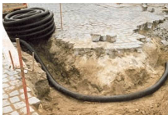
Kabuflex R and Kabuflex R-UV – provide advantages in inaccessible terrain and on uneven ground
