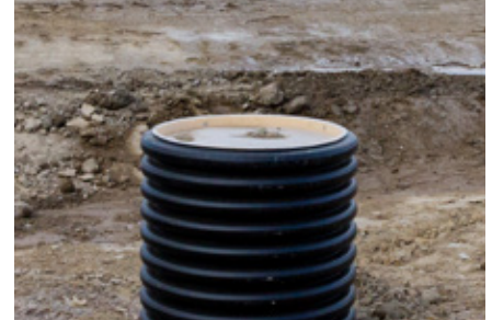
Temporary construction site cover for extension pipes
