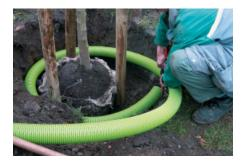
The totally perforated tree preservation pipe is installed as a loop in the root zone under the throughfall and connects to a tee.
