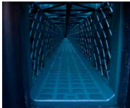
The inspection camera goes from QuadroControl directly into the inspection tunnel of Rigofill inspect
