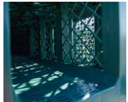
Large openings in the side wall of the tunnel
